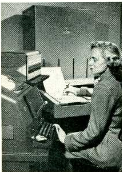
Large cabinet (left) is space-control unit, heart of Intelix system being installed by Penn. R.R. Operator receives on the teleprinter a coded message from a ticket seller for a reservation. Unit automatically selects from trays in cabinet the one containing car diagrams for trains on day requested. Operator selects proper diagram and flashes back confirmation. At right is one-sixth of the behind-the-scenes brain of the Intelix system. Gas triodes, shown at immediate left of engineer, convert incoming teleprinter characters into currents that actuate appropriate relays to bring desired tray file in front of operator at left
