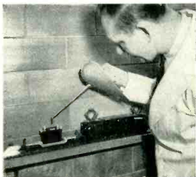
Radioactive chemicals are carried between rooms by a toy electric train
